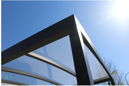
Transparent: 80-90% transmission de lumière
