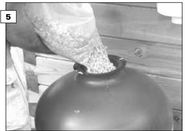
5 Fill the filter first with gravel (3-5mm) and then with sand (0.4-0.8mm). The sand has an unlimited lifetime and only need to be topped up in case sand is lost. Mark the level of sand/gravel to be able to re-fill the filter to the correct level at a later time.
