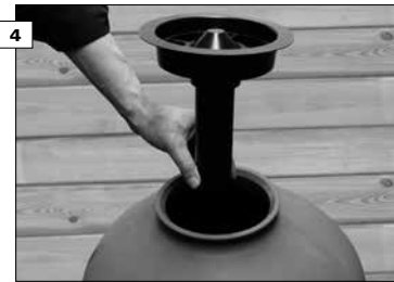
4 Make sure that the plastic protection (funnel) is placed on top of the filter to prevent sand/gravel from falling into the mouthpiece of the branch pipe.
